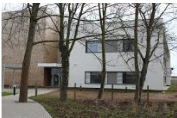
HARC’s main entrance with the public block on the right
